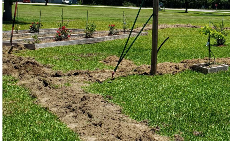
Completed underground and auto-timed irrigation system at pollinator garden
