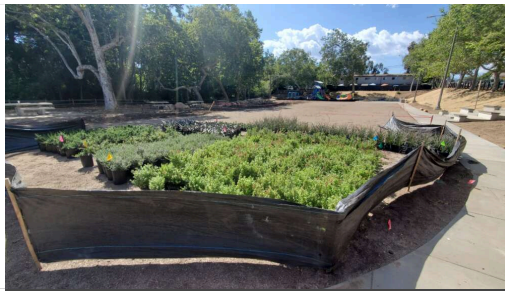
Bohnett Park Plant Staging
