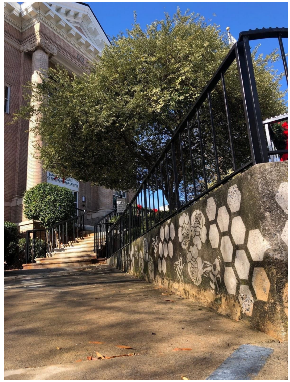
Clean Graffiti outside City of Gastonia municipal building - completed by using a stencil and powerwashing
