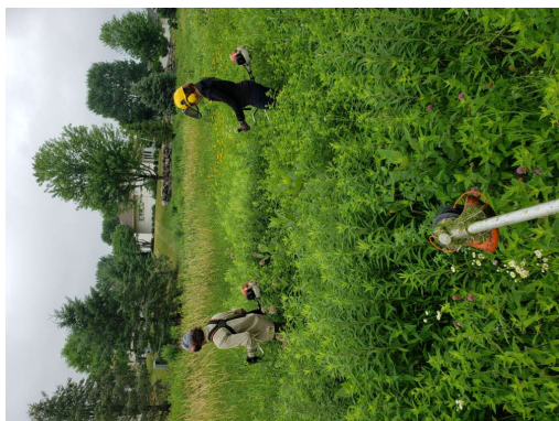
Brush mowing to control invasive reed canary grass in a prairie stormwater retention pond
