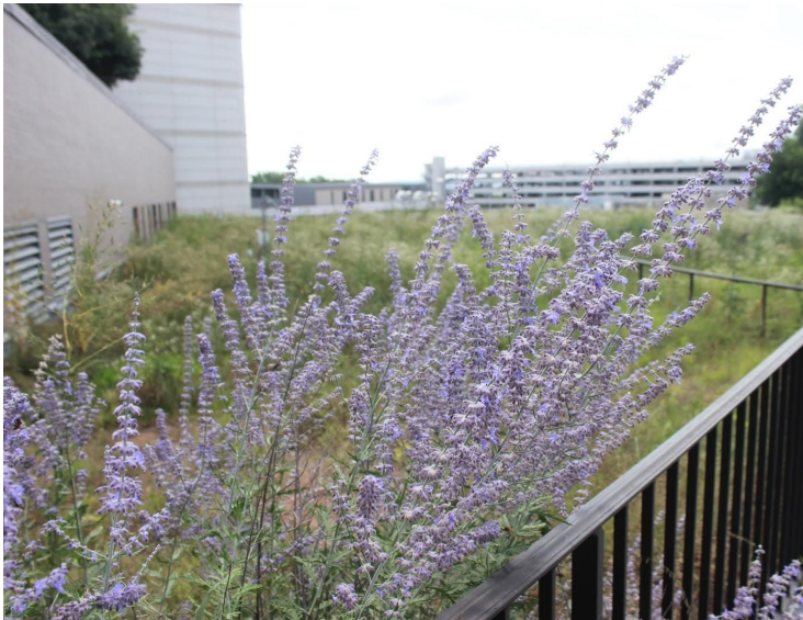
Russian Purple Sage growing on the Hillside Auditorium Green Roof.
