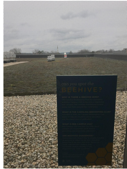
Permanent signage on the Fed Ex Global Education Center educating classes who meet in this space about the beehives on the green roof that are maintained by the Carolina Beekeeping Club. You can see the hives in the background!
